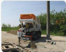
ZS1260 on the job site
